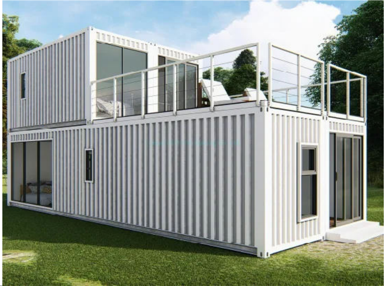
RESIDENTIAL CONTAINER POLAND
